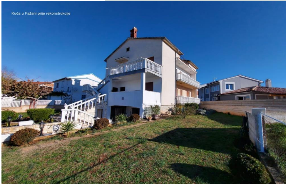
Before the reconstruction
