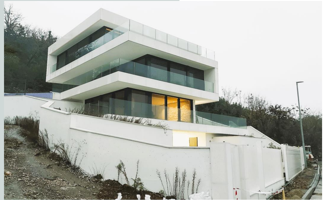
Construction site, almost finished
